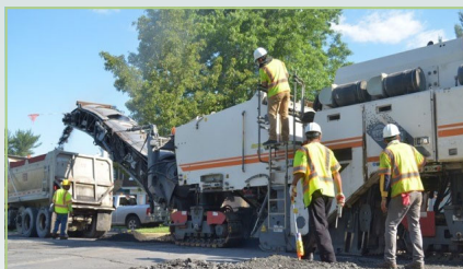
Typical milling operation
