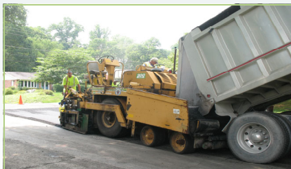
Typical hot mix asphalt paving operation
